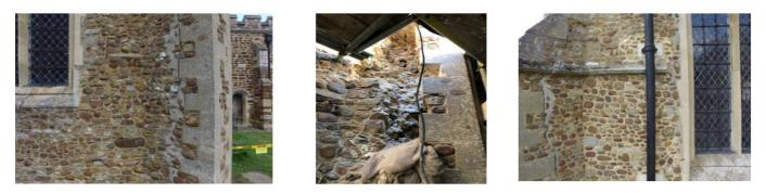
The work required here was extensive and all the damp damaged, crumbling mortar had to be removed before reinforcing internal steels were added to tie the buttresses back to the body of the building. Earlier repairs using cement instead of lime mortar had not solved the problem.
