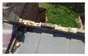
Stonemasons carved local matching stone to replace those which could not be conserved. The new lime mortar is to match the original (seen in the background of the outer nave wall) not the cement mortar of earlier repairs (seen below the current restoration works).
