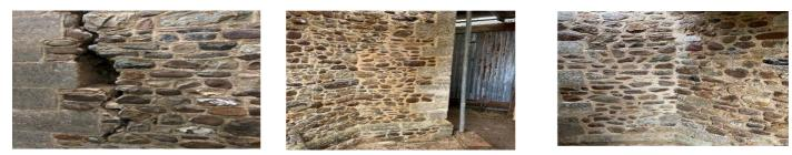
The final repairs don't tell the story of how much work was done here. All the original stonework was salvaged and conserved. Great care was taken by our Architect and the Contractor to get lime mortar mix that matches the original lime mortar in both colour and texture.
