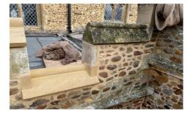
Buttresses at the south side of the church were unstable and urgent repair works needed. Rather than supporting the building it was the building keeping the buttresses standing - just.
