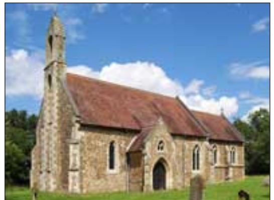
▼ St Denis' church today: a handsome building now owned by the Friends of Friendless Churches, which is safeguarding it in perpetuity.
